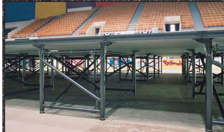
Large open spaces beneath the decks are ideal for stringing cables or stage-side storage.
